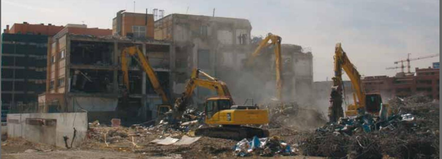
Construction management of all kinds of mechanical demolitions using our own and special machines for demolitions, long reach arms, hydraulic breakers, hydraulic shears and heavy duty hydraulic hammers.
